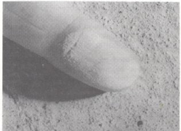
Dusting concrete surface.
