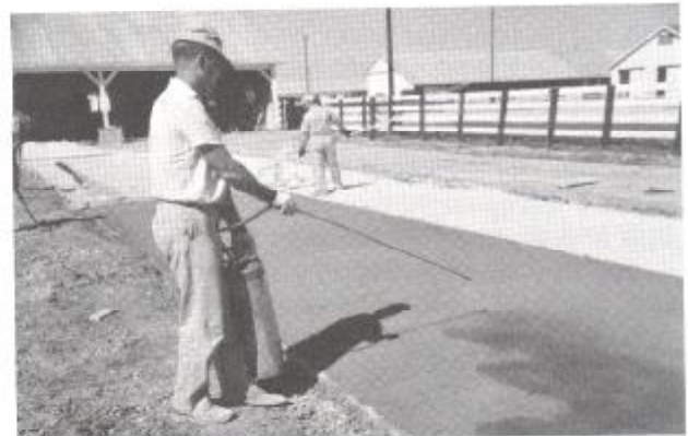
Application of liquid membrane-forming compound with hand sprayer.
