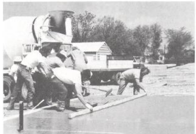
Finishing Concrete Flatwork
